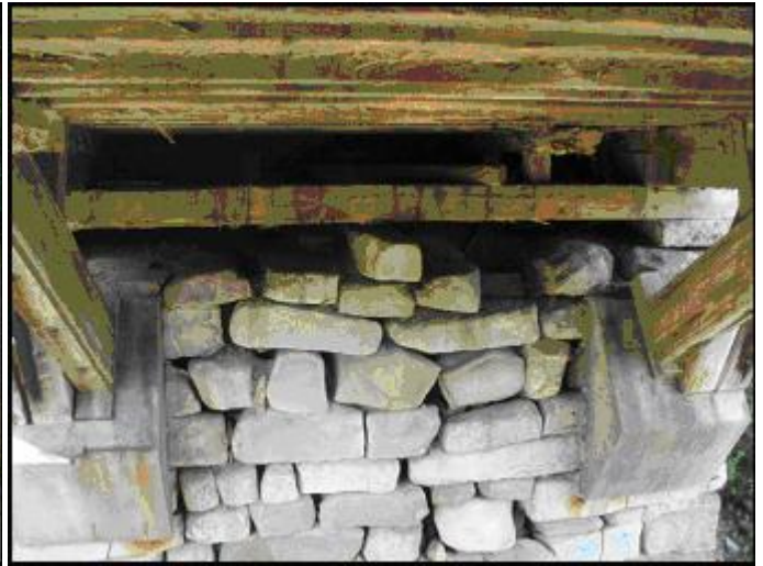
Voids and Settlement in the Stone Pier and Abutments
