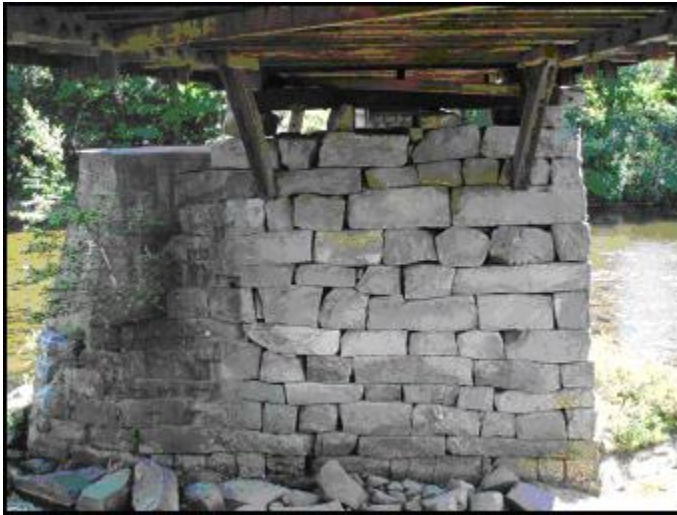
Voids and Settlement in the Stone Pier and Abutments
