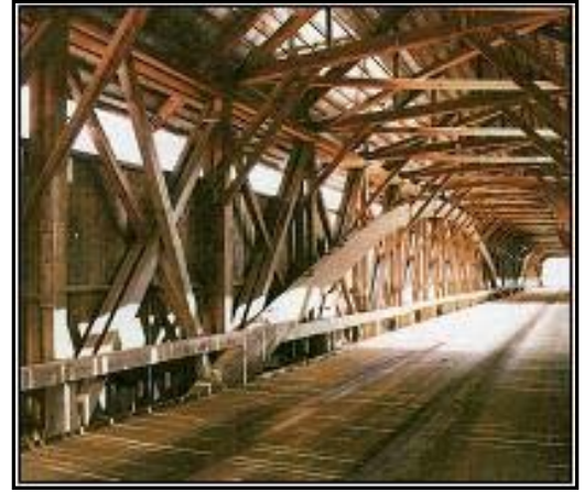
View of Truss Interior
